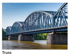
A truss bridge is built from triangles called trusses. Triangles are the strongest shapes, so this bridge can carry heavy weights.
