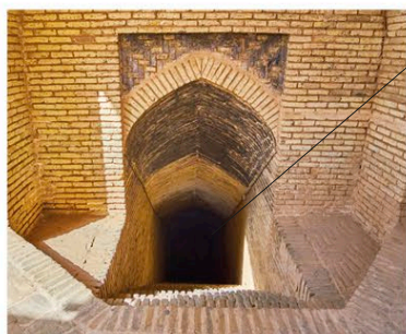
QANAT (IRRIGATION SYSTEM) The underground qanat tunnels brought water from freshwater sources to the farms.
